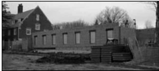
The Barker Hall addition in progress and on schedule.
